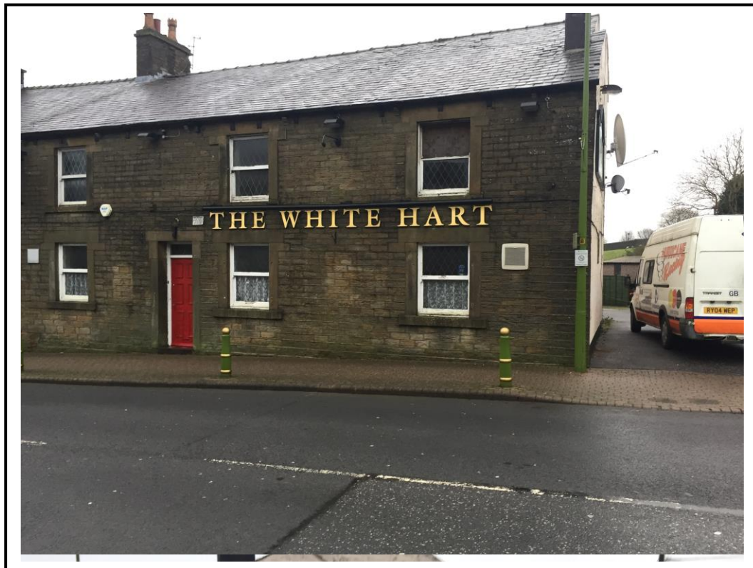
Photo 1 – front elevation of existing building
